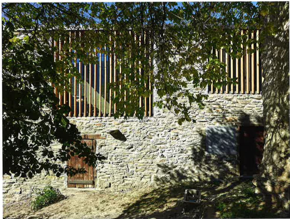
(Above) The rubble masonry moves downhill with the natural gradient of the land. The design retained existing openings on the ground floor, with wooden screens installed above.
