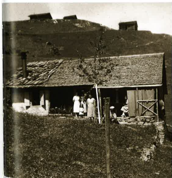
(Right) The home is perforated, which separates the timber and masonry sections. This reinforces the transverse effect and minimizes the need for other openings in the outer walls.
